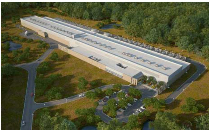
Facebook data center in North Carolina
