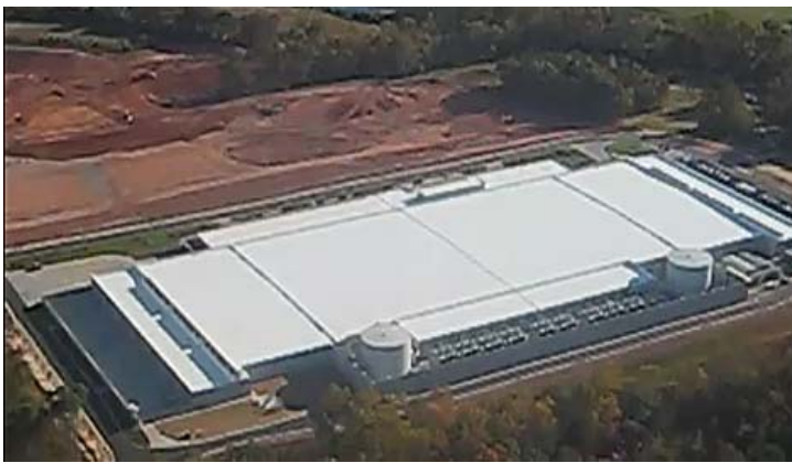
Apple data center in Maiden, North Carolina
